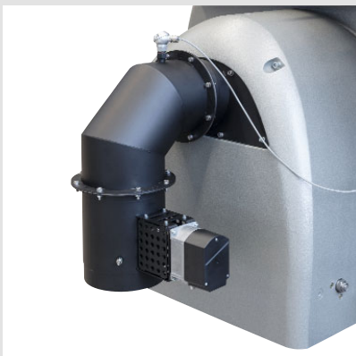
FGR connecting bend with actuator and Pt100
