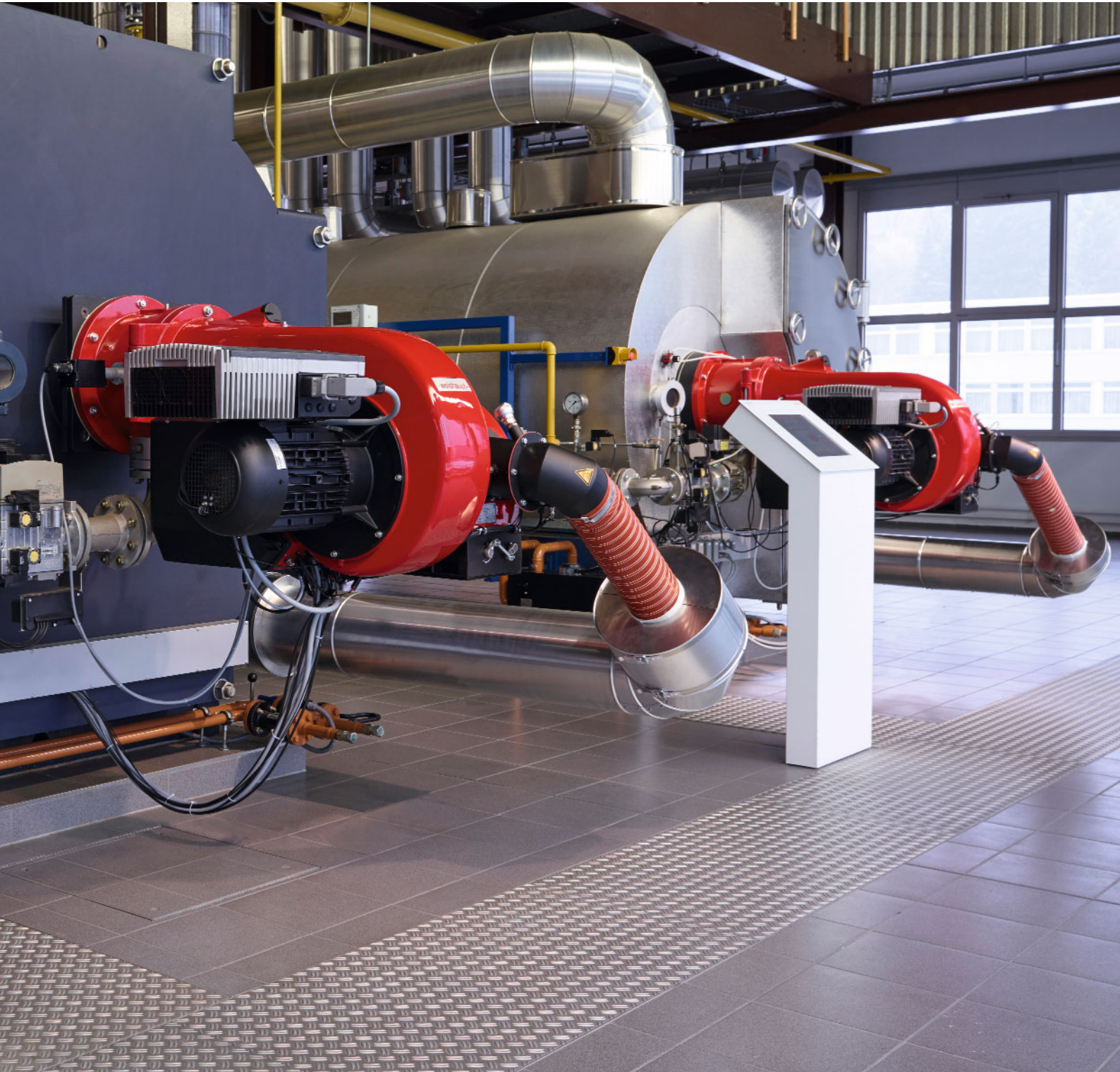
Burners with FGR on long-term test in the Weishaupt factory's boiler room
