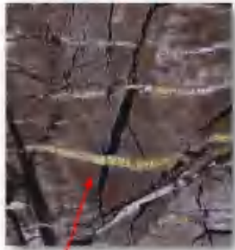
局部实拍 Detail in part
