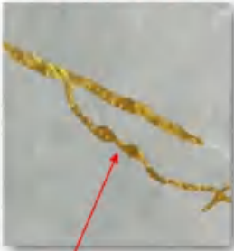
局部实拍 Detail in part
